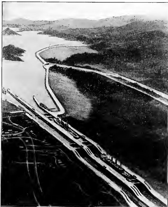
BIRD'S EYE VIEW OF GATUN DAM
